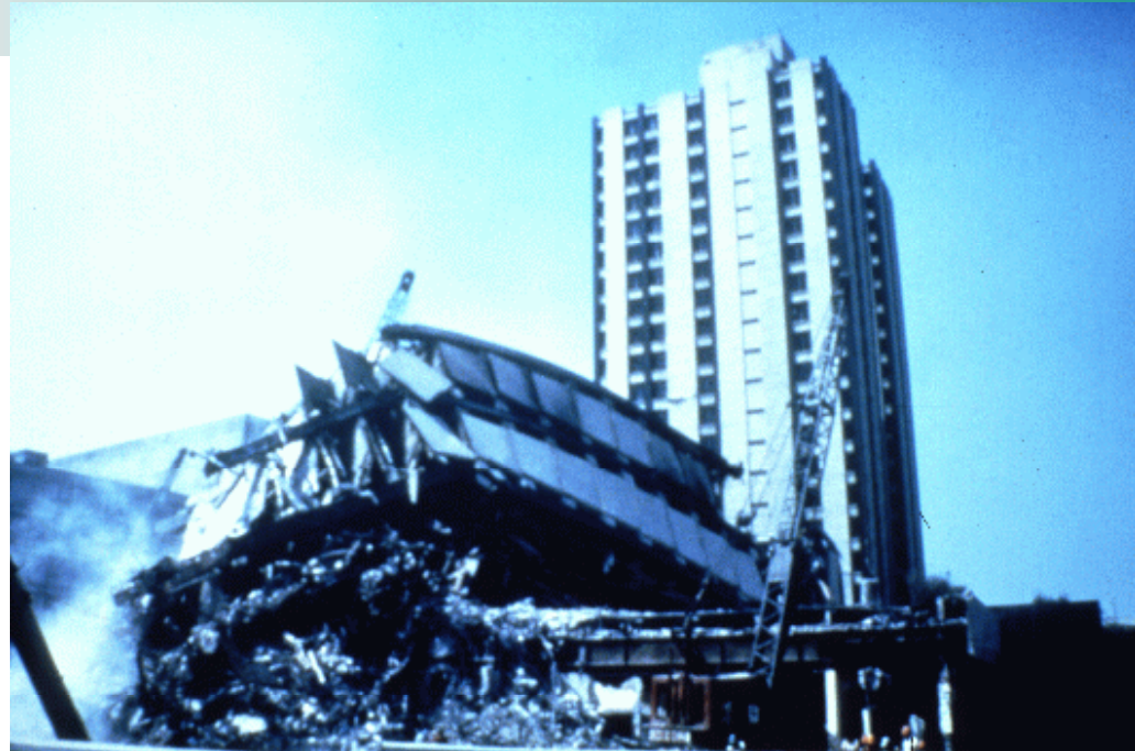
Collapsed 21-Story Office Building. Buildings such as the one standing in the background met building code requirements
